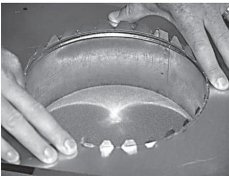
**Step 3.** Press down firmly on the sheet metal plenum. Lock the collar in position by bending the collar tabs outwards and flatten
