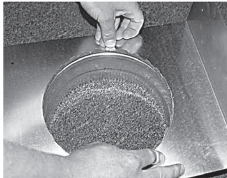
**Step 4.** All collar tabs are flattened. Repeat steps 1 – 4 for top duct assembly.
