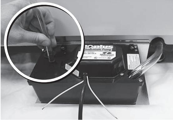
**Plug in the condensate pump and the assembly is completed.**
