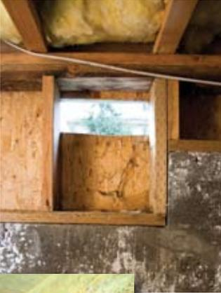
Mold growth on crawlspace foundation beams.
