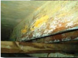
High humidity in a crawlspace can lead to wood rot and buckled hardwood flooring.
